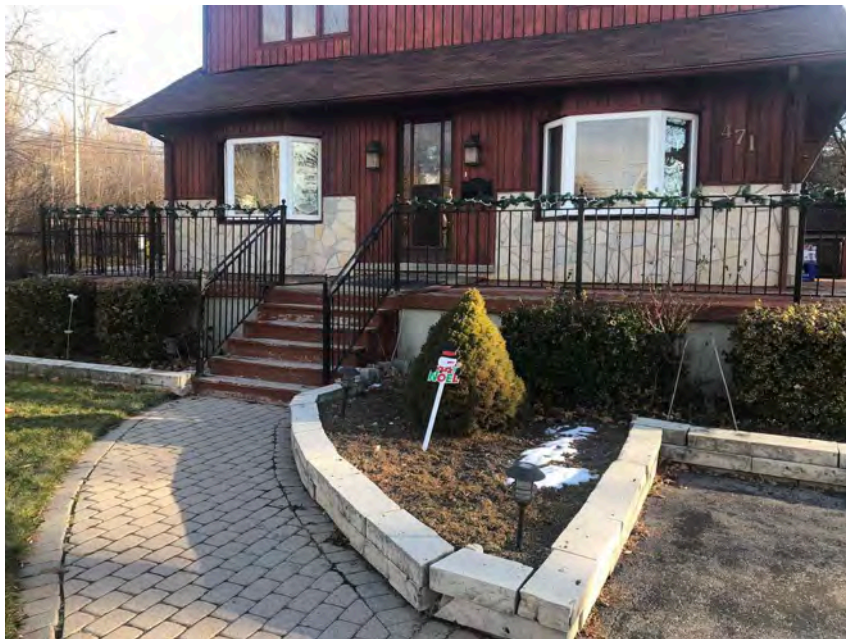
Plate 10; Shows condition at the time of field Survey.
