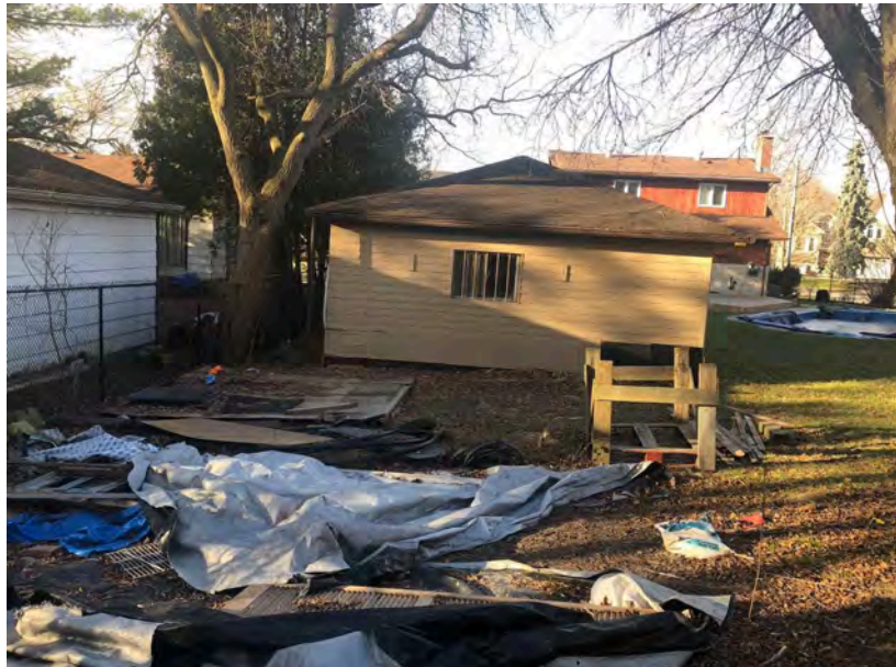
Plate 4 Shows condition at the time of field Survey.
