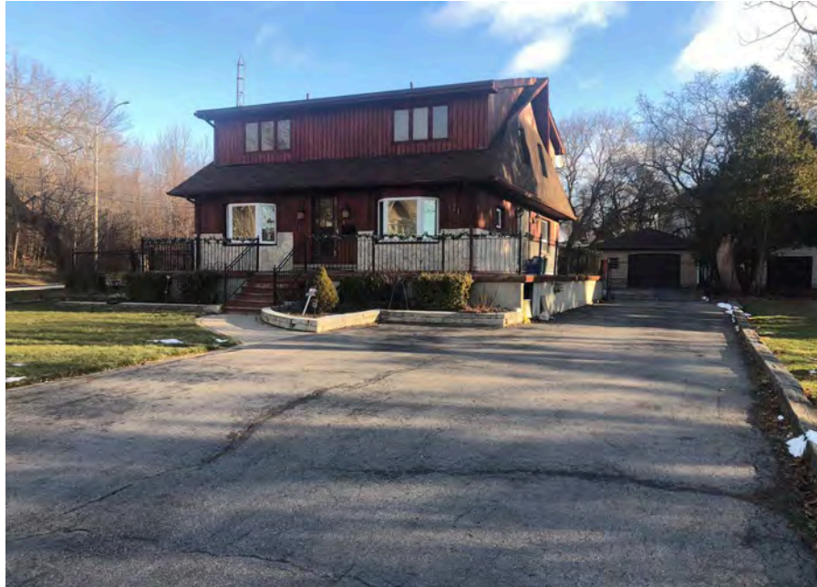
Plate 7 Shows condition at the time of field Survey.
