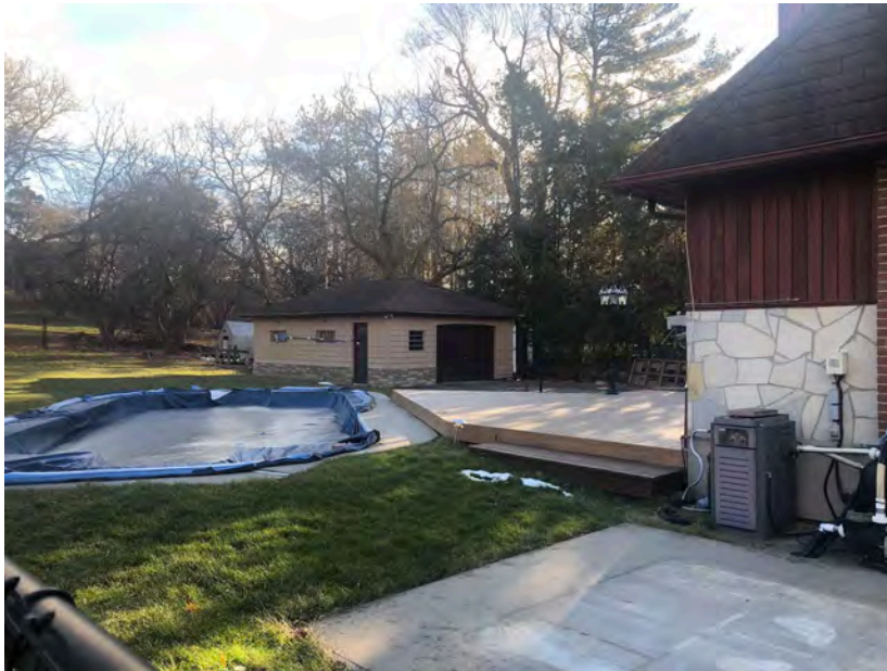
Plate 6 Shows condition at the time of field Survey.
