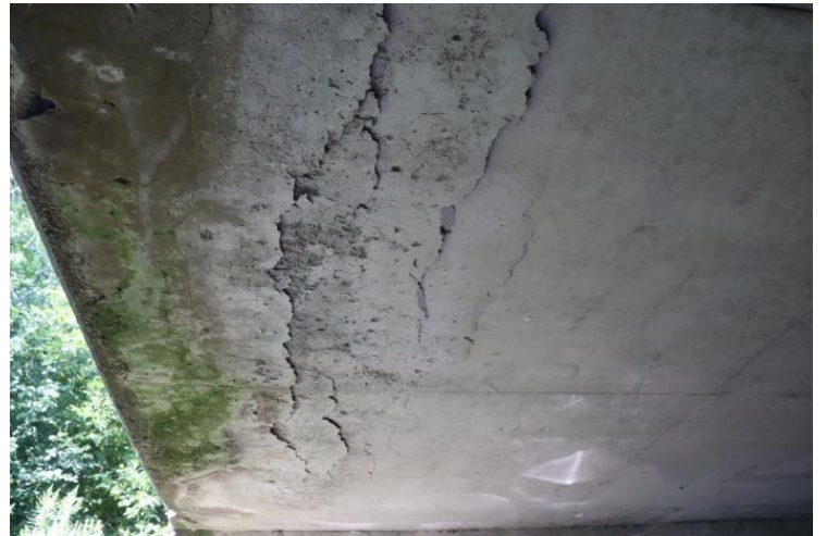
Image 4: Delamination in the bridge structure
