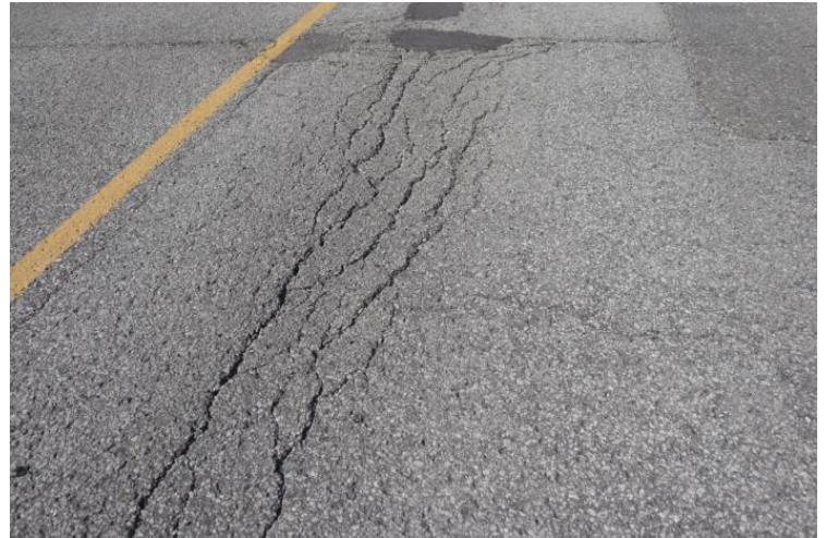
Image 2: Cracks in the pavement
