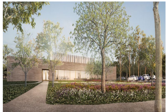
Net zero community infrastructure project
