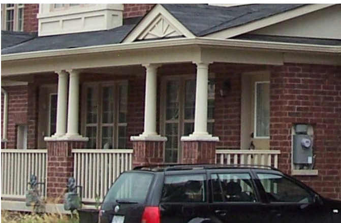
Examples of screening of mechanical equipment
