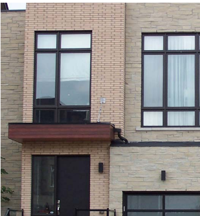
Examples of exterior building materials
