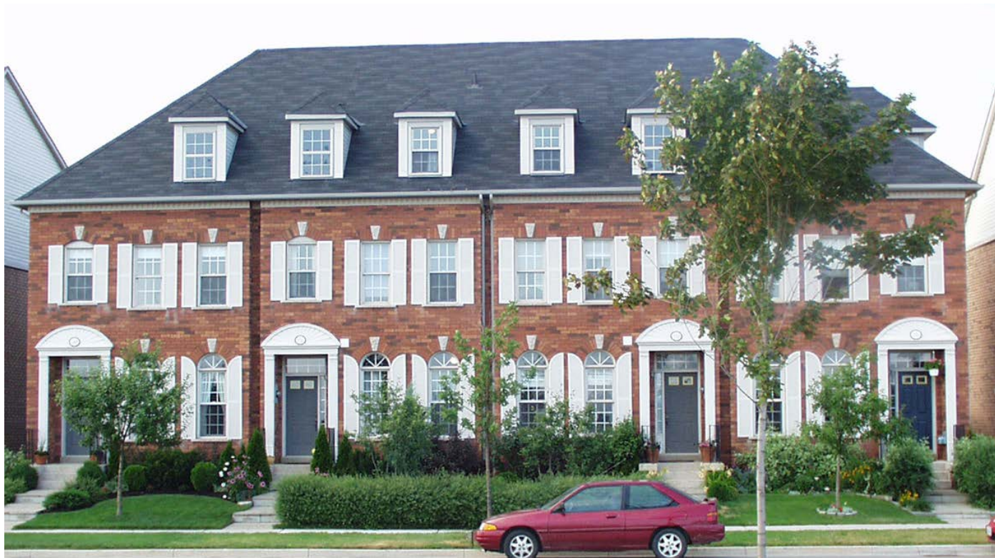
Example of a streetscape with a traditional architectural style
