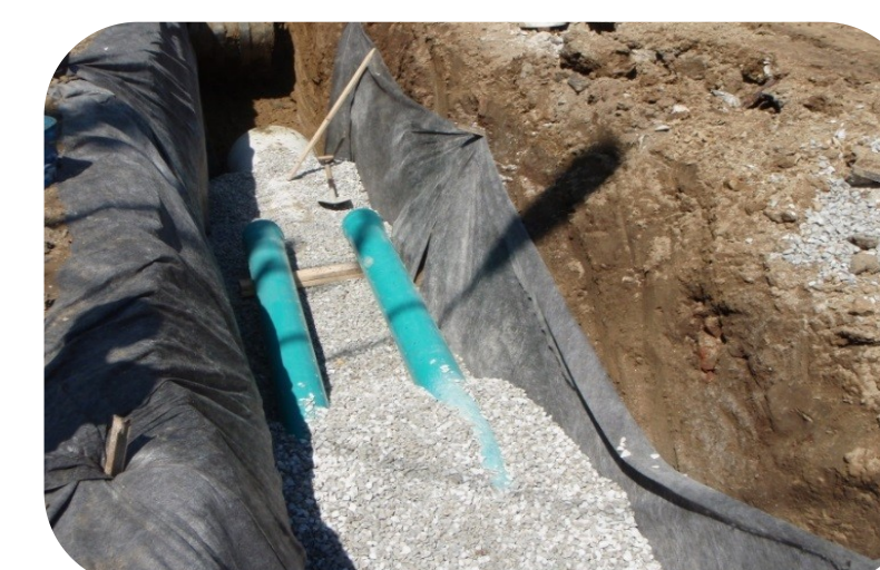
Perforated Pipe System
