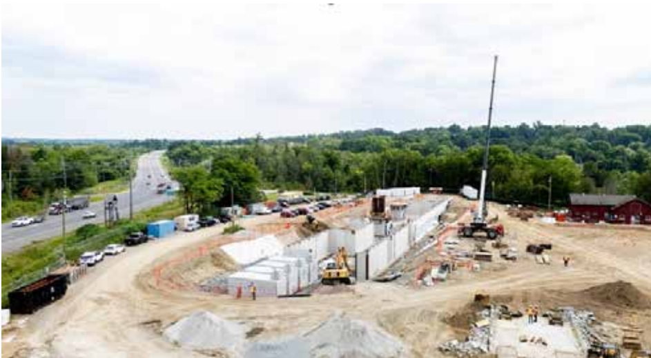
Summer, 2024 – the foundation of the facility and concrete placement of foundation walls is complete
