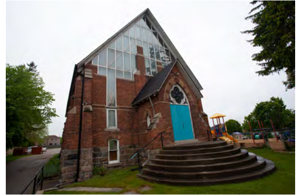
11. Primary (south) facade, shown from a southwest angle to reveal the blend of 1877 masonry and 1974 glass.
