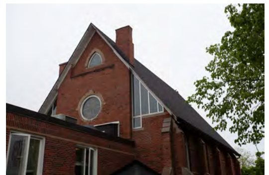
15. Rear (north) facade, showing Baird’s intervention, albeit to a lesser extent, alongside the “1974 Addition.”
