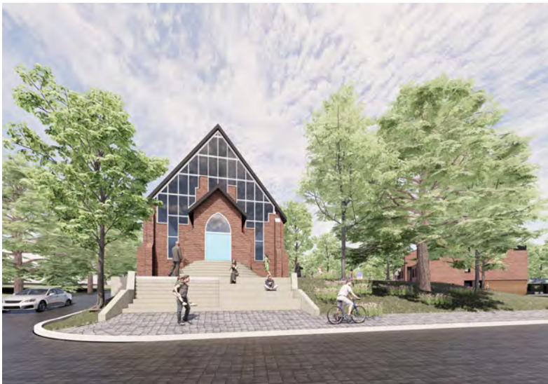
107. Render of the retained 1877 Church (as rehabilitated in 1974). Note the proposed development's intention to reassess the retaining wall to allow the Church building to communicate openly, once again, with Dunbarton Road. (KPMB, 2022).
