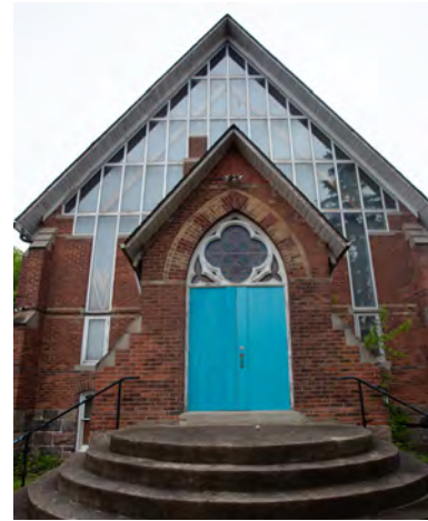
77. South elevation of entrance vestibule, chapel building.
