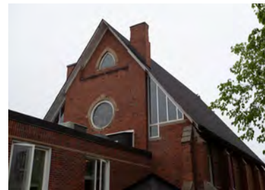
76. North elevation of the chapel building.
