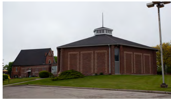
92. Overall building, as viewed from NE.
