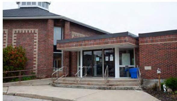
97. West entrance to 1974-1985 addition.
