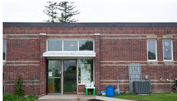
94. East entrance to 1974-1985 addition.
