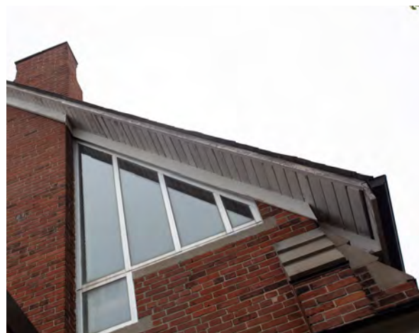
91. Curtain wall assembly at north elevation, chapel building.
