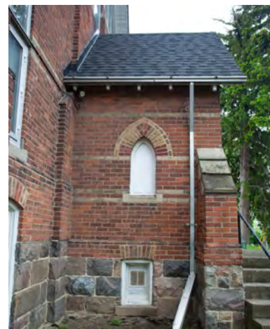
78. West elevation of entrance vestibule, chapel building.
