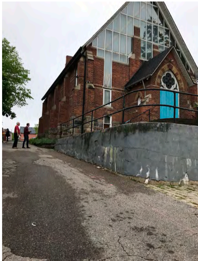
31. Southwest view of the 1877 Church. Note the existing driveway access to its west, and the concrete retaining wall that now disconnects the building from the historic thoroughfare.
