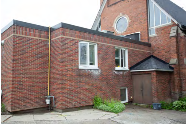
18. Rear (North) facade, showing part of Baird's "1974 Addition."
