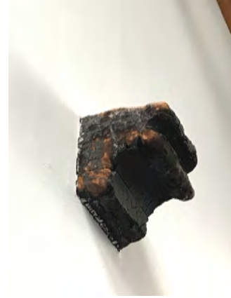
19. Charred timber left in situ during Baird's Post-Modernist rehabilitation.
