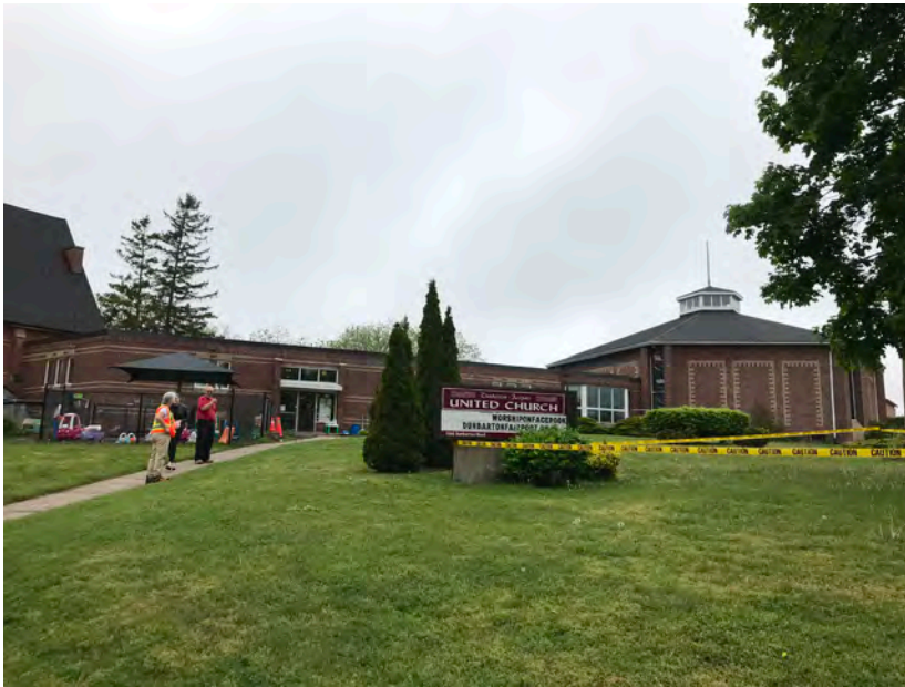
20. Southeast view across the lawn, revealing the "1985 Addition" of rectilinear spaces matching the scale and character of the "1974 Addition," along with the more prominent octagonal sanctuary space.
