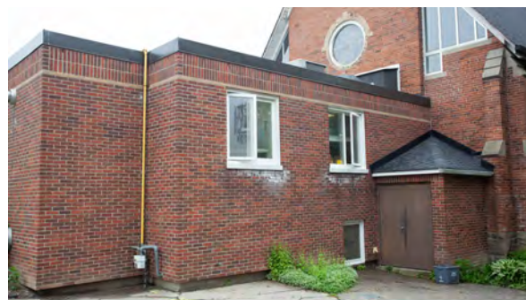
100. Southwest portion of 1974-1985 addition, adjacent to north elevation of chapel building.
