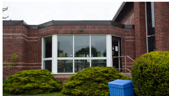
95. Bay window at east elevation of 1974-1985 addition.
