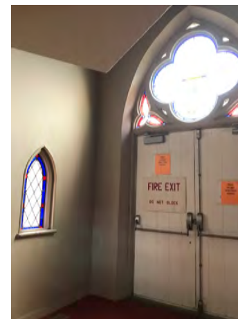
13. Interior of Primary (south) facade porch, revealing original remaining glass encased in contemporary walls.
