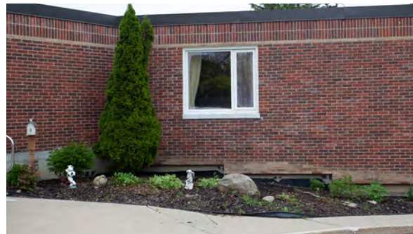
98. New garden bed south of the west entrance to 1974-1985 addition.
