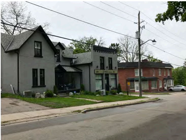
48. Southwest view towards the intersection of Dunbarton and Dunchurch Roads, showing the former home/shop of Sadler, and the former Lynde & Son shop.
