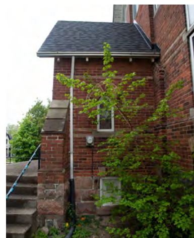
79. East elevation of entrance vestibule, chapel building.
