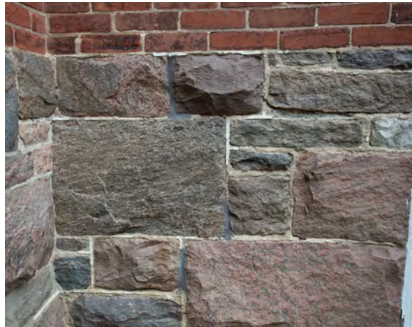
83. Typical condition of cut stone base.
