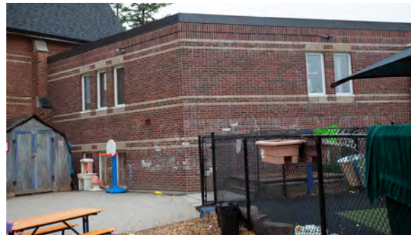
93. East elevation of 1974-1985 addition.
