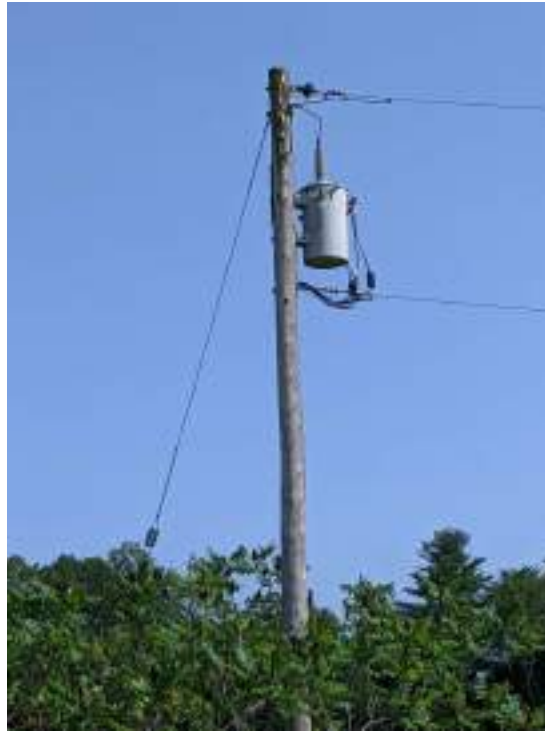
Site Photo 9. Transformer located on a telephone pole in the western portion of the Site. No spills, staining, discoloration or leaks observed.
