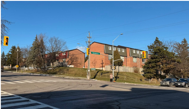
Looking northeast toward existing three storey townhouse development from southwest corner of the intersection at Liverpool Road and Glenanna Road.
