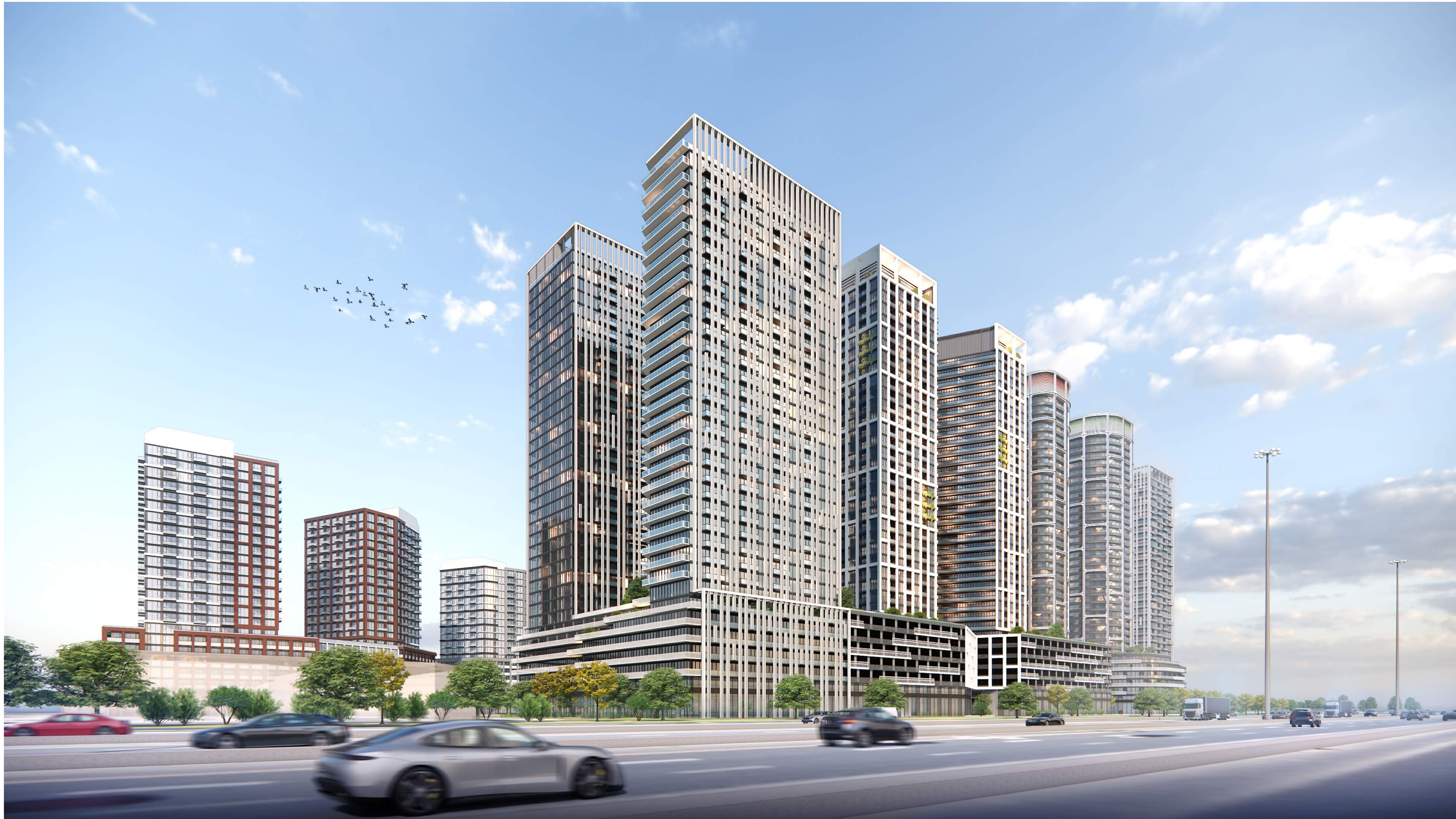
VIEW FROM THE KING'S HIGHWAY NO.401 LOOKING NORTHEAST
