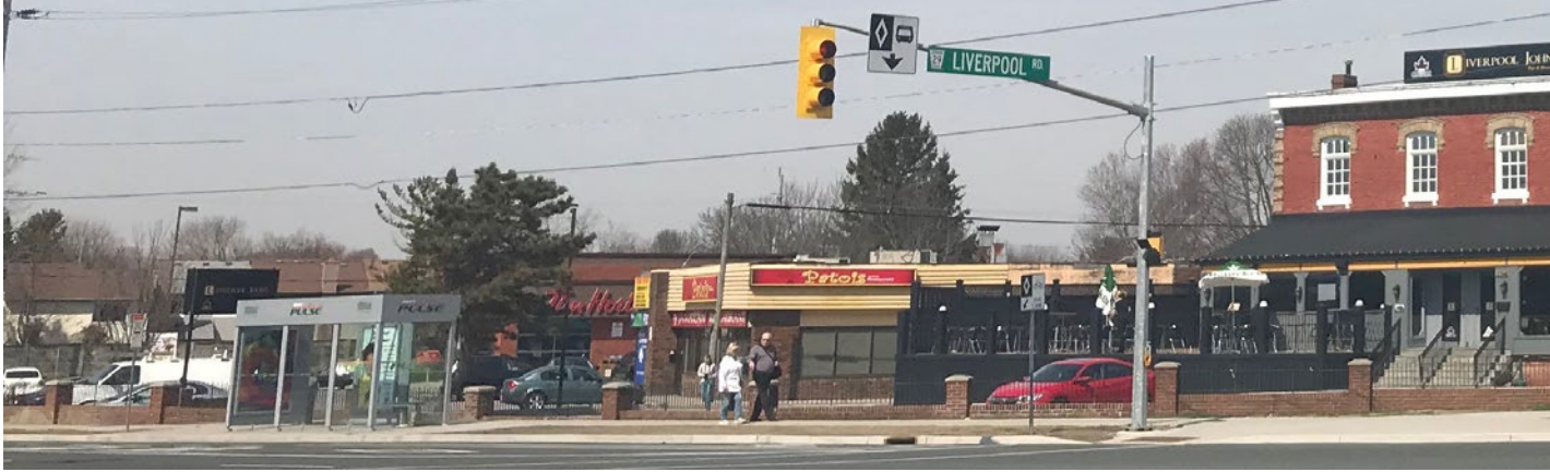
View to the Old Liverpool House from the southeast corner of Kingston and Liverpool Roads (ERA, 2018)
