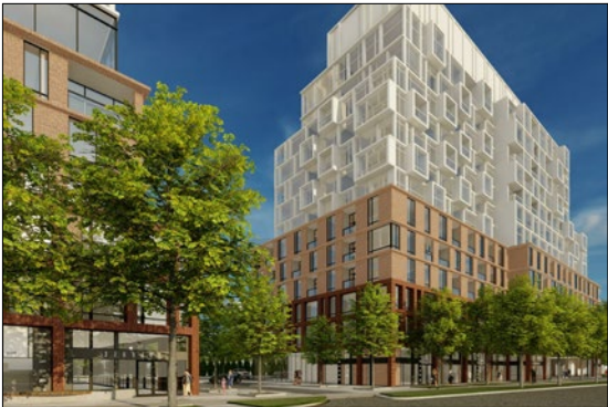
View of Building A from the southeast 5 26.2
