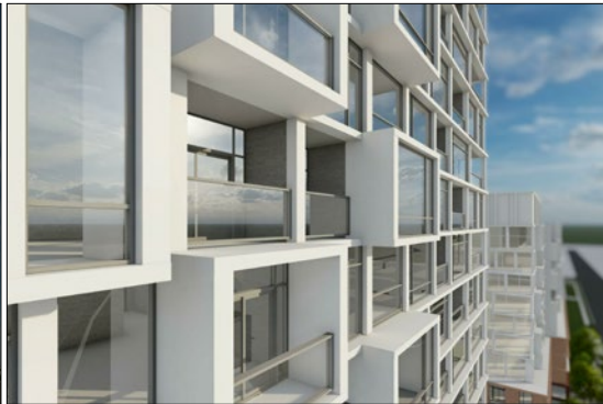
View of lower facade detail 11 28.1
