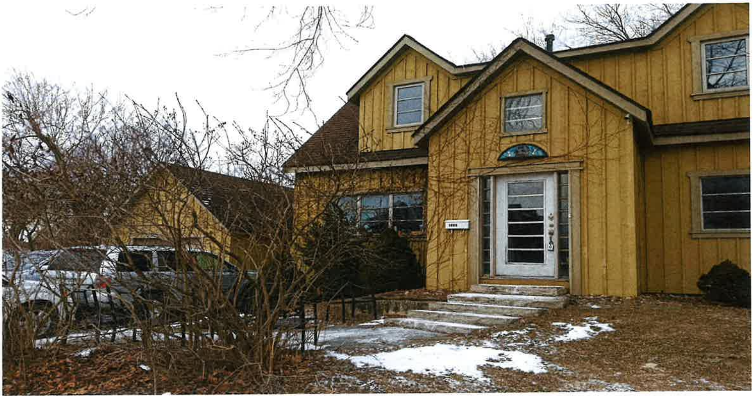
General view of the entrance at 1885 Glendale Drive in the western portion of the subject site (looking northwest)
