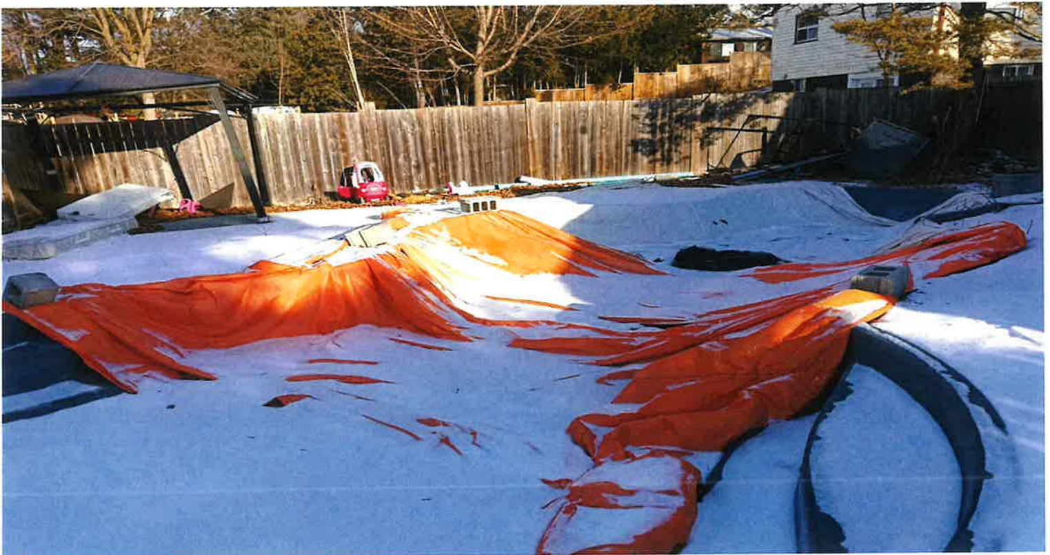
General view of the pool (currently not in-use) in the northern portion of the subject site at 1884 Liverpool Road (looking north)
